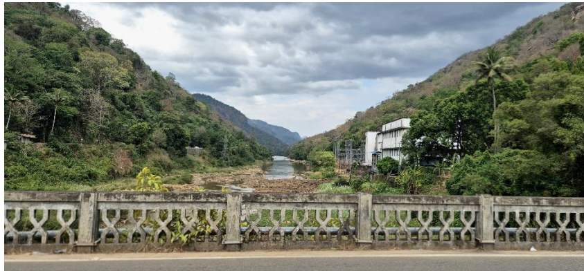
Figure 23(c): Photograph showing the confined valley setting near Panamkutty Bridge
