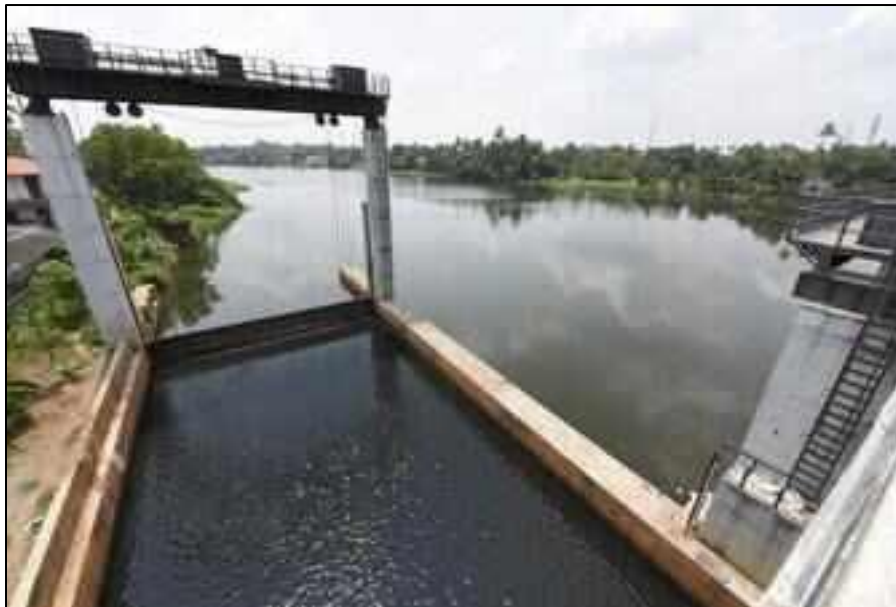
Figure 2: Discolored river water at KWA intake disrupting water supply at Aluva and Chembaracky ( Source: Times of India )
